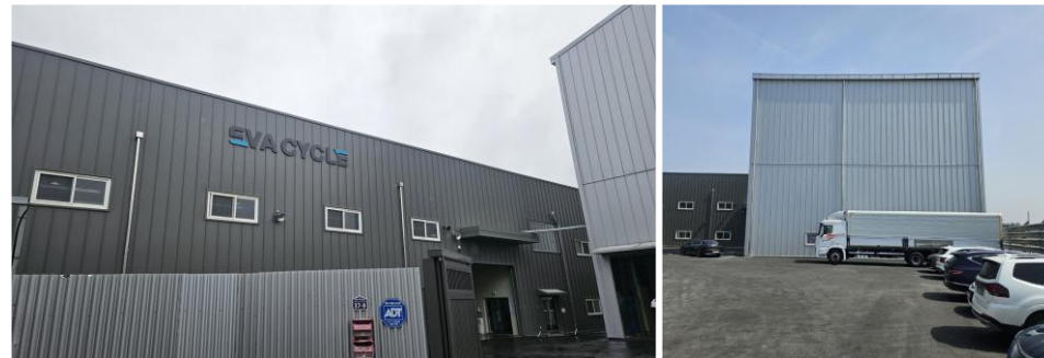
[ View of Works ] Hwaseong 1 works
